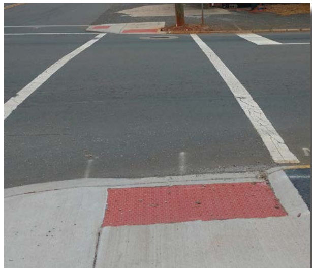
Below: A good example of ADA-compliant curb ramps recently installed at the Gold Street/Main Street intersection in downtown New London.
